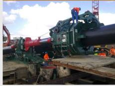
For the Westerwoldsche AA and Wymeerer Sieltief river crossing the company decided to use an Herrecknect 750ton pipe thruster. Due to the very soft and muddy soil conditions, the installation required a temporary basament with 16 1000mm pipes driven in the soil and a complex system of steel beams to support the pipe thruste, to be built in less than 10 days.
