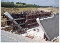
In 2010 a 2km bypass connecting Sp46 to SP588 near Busseto, Province of Parma. A concrete monolithic underpass was needed to pass the RFI Fidenza-Cremona railway.
