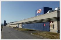
GTE is Barilla's main civil engineering consultant for the 28200 sqm plant of Rubbiano. After the 2012 earthquake, the Company started the seismic retrofitting of the plant in order to increase safety to 60% of the design seismic load for this region.
