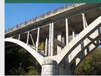
Lamberti Bridge is a 3 arches Maillard type concrete structure on a main road in the Province of Parma. Built in 1933 it now needs a seismic retrofit and structural restoration.
