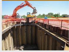
The 1200mm natural gas pipeline, designed to strengthen one of the most important gas networks in the North of Italy, has a lenght of 85 km and a working pressure of 75 bars. Several *trenchless* technologies such as minitunnels, controlled horizontal drilling and direct pipes were adopted.
