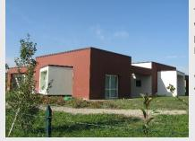
The structure of this building is made by PlastBau walls. These stay in place EPS formork include a prefabricated reinforcing bar system. Class A Energy building
