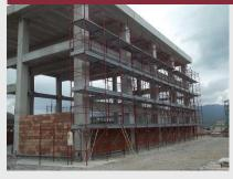
The Montesano Snam Plant is located in the highest seismic level of Italy. Overstructure is a concrete prefab frame, foundations are cast in place footings over a pile-consolidated soil.
